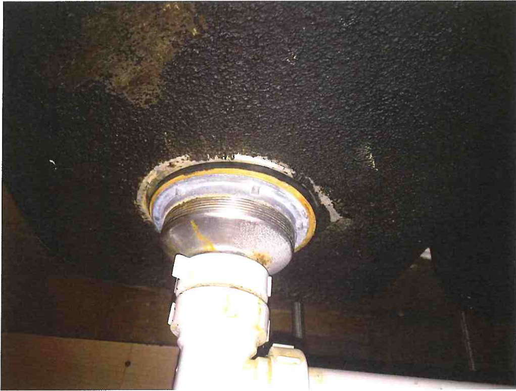
Asbestos Containing Sink Undercoat (Black), Kitchen
