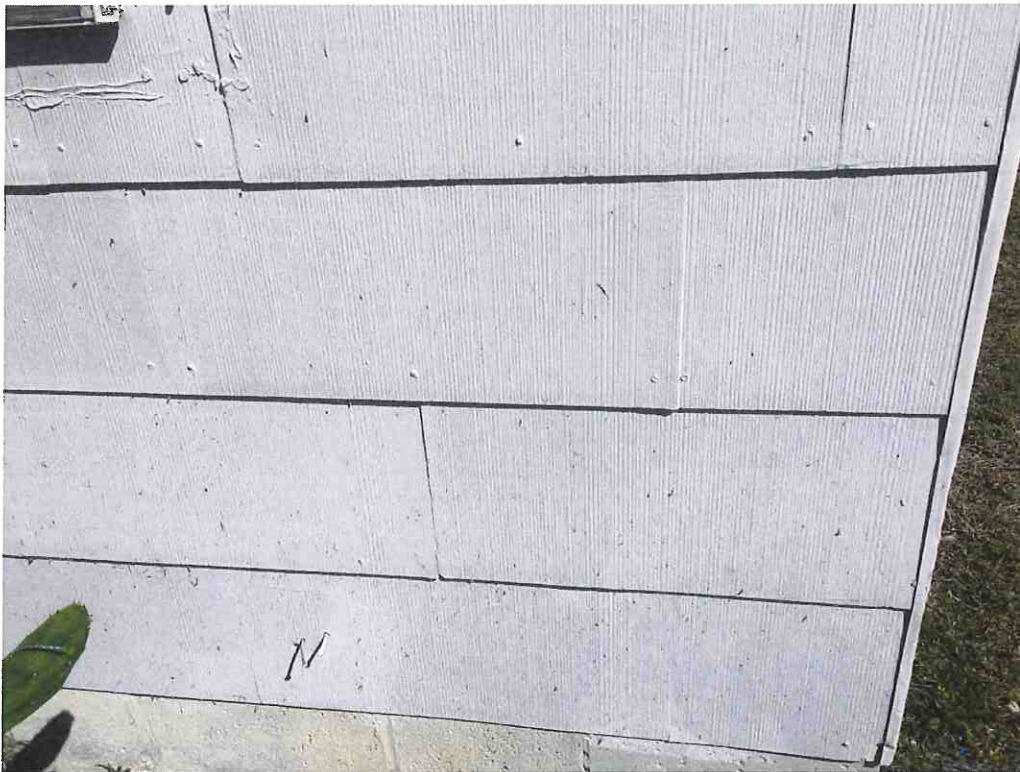
Asbestos Containing Exterior Transite Siding, throughout Exterior
